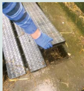
Close slurry openings.
