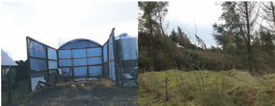
Some damage to sheds and land caused by Storm Darwin.
